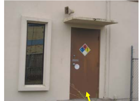
Figure 17 Rear entry door
