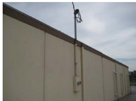
Figure 4 Single phase overhead Electrical service
