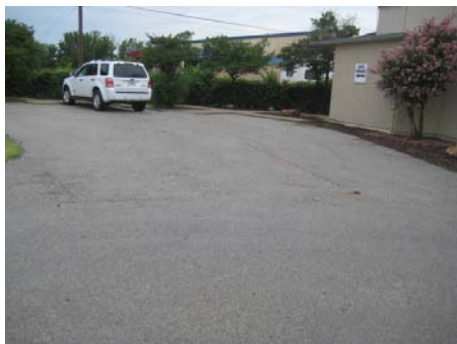
Figure 1 Front parking area
