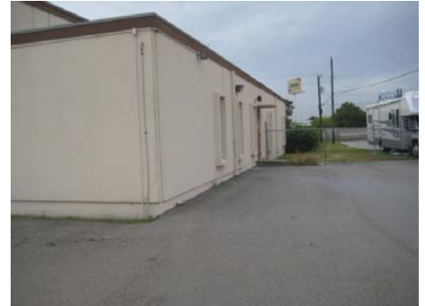
Figure 8 West side of building
