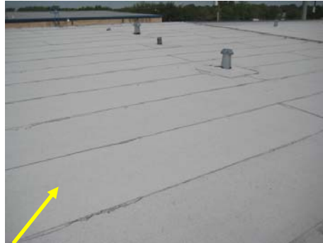
Figure 28 Modified Bitumen-SE to NW view
