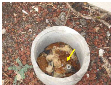
Figure 14 Missing handle at front hose connection
