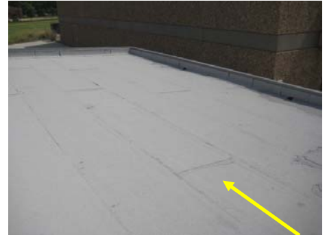
Figure 29 Modified Bitumen-South to North view
