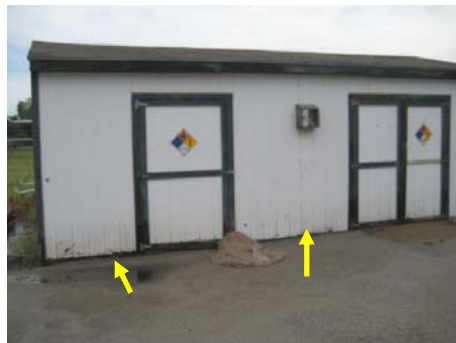
Figure 20 Storage building-property rear
