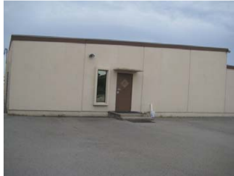
Figure 7 North side of building
