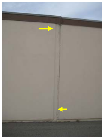
Expansion joint-East side.
