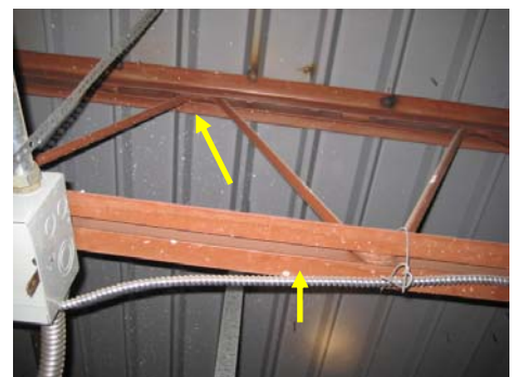
Figure 27 Metal trusses-attic example
