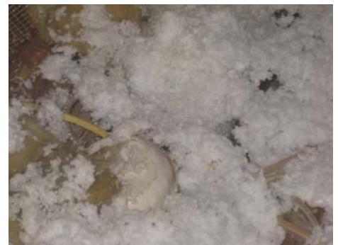
Figure 22 Recessed lights touching insulation
