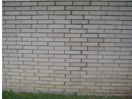
Figure 7 Repaired mortar cracks-West side of garage
