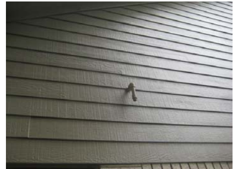
Figure 10 West side auxiliary drain runs when AC runs
