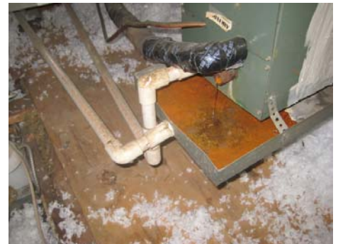
Figure 20 East AC unit-pan holds water
