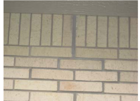
Figure 8 Repaired mortar cracks-West side of garage
