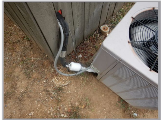
The Air Conditioning System has icing of the evaporator coil/ suction line at some of the units. (Approximately 4 were observed) Recommend further examination and repair as needed.
