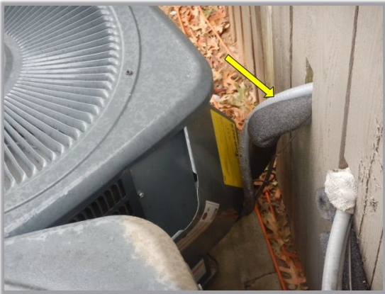
The Air Conditioning System has icing of the evaporator coil/ suction line at some of the units. (Approximately 4 were observed) Recommend further examination and repair as needed.
