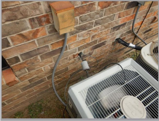
Damaged conduit at some of the AC condensers. Recommend repair or replacement as needed.
