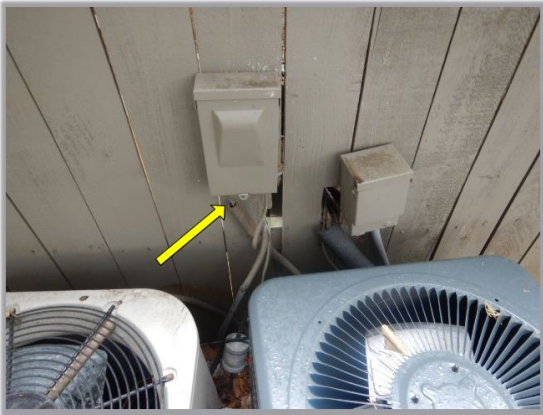
Damaged conduit at some of the AC condensers. Recommend repair or replacement as needed.
