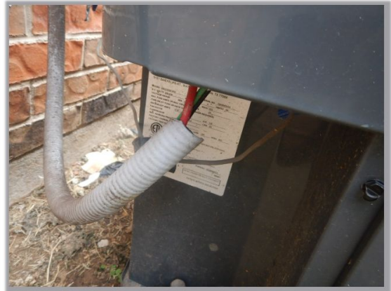
Damaged conduit at some of the AC condensers. Recommend repair or replacement as needed.
