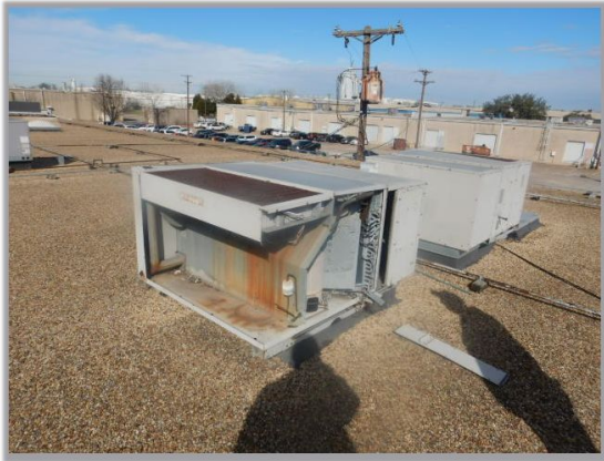
Package unit with Electric AC and Gas furnace Unit #18 GE
