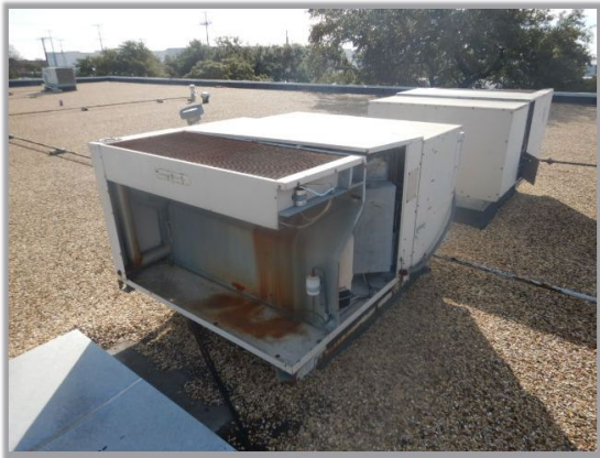
Package unit with Electric AC and Gas furnace Unit #19 GE
